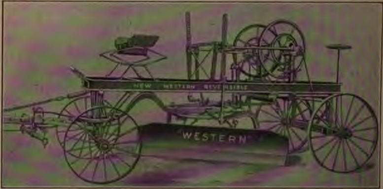
Standard Road Grader. Figure 12.
